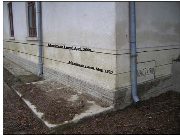
Figure 3. Bechet Harbour Building, with the marks of 1970 and 2006 floods (photo by Boengiu S.).
